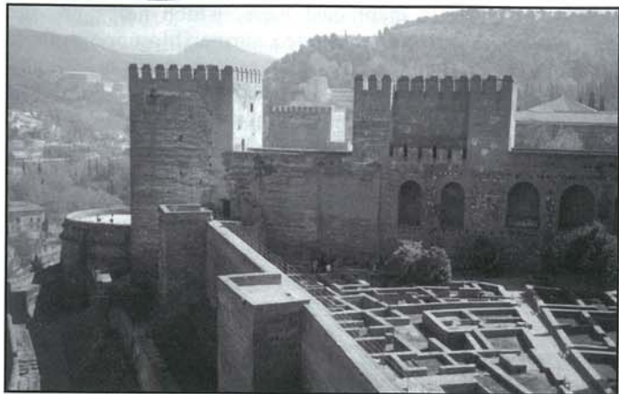
The Alhambra castle-citadel, built atop the highest hill in the city of Granada by the Moors, starting in the 7th century, is a must-see.
